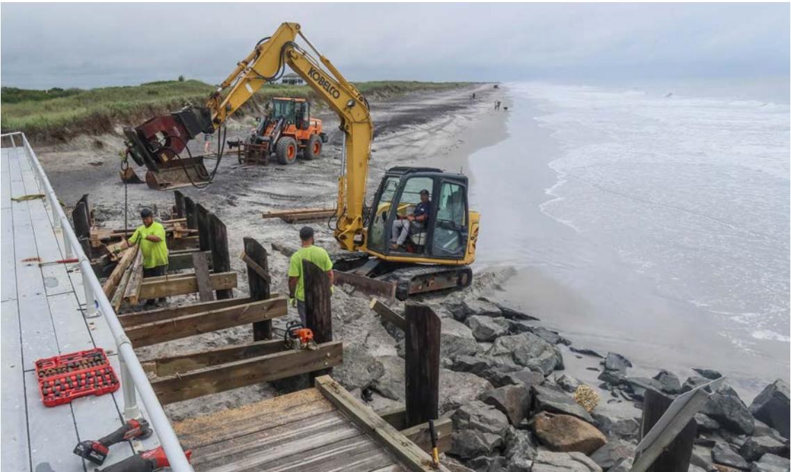
Demolition moves forward at the Promenade’s North End Beach Access Ramp on August 17, 2026. The city of Brigantine has been working with Atlantic County (which is responsible for the promenade) to ensure that work on the sea wall is appropriately completed. (Photo by Sean Kardon).
