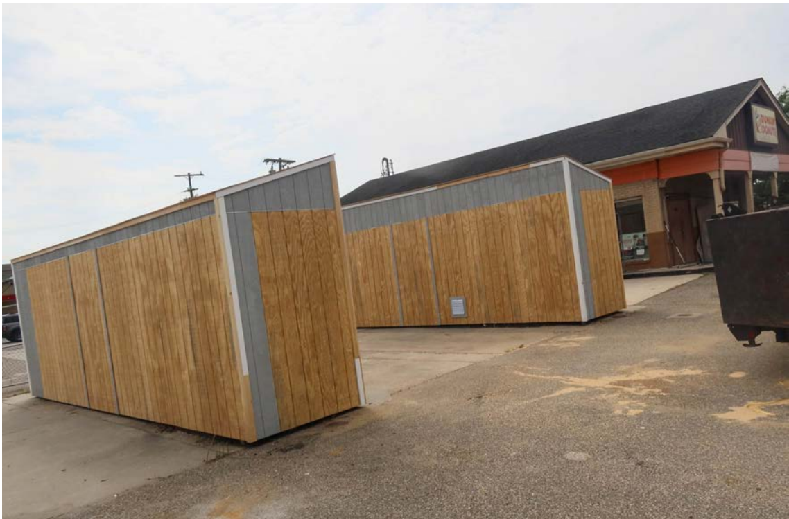
Demolition is nearly complete of the canopy at the closed Conoco Gas Station that is connected to the Dunkin Donuts has begun at the corner of Brigantine Boulevard and Harbor Beach Boulevard, and the old pumps have been closed in for the time being. (Photo by Sean Kardon).
