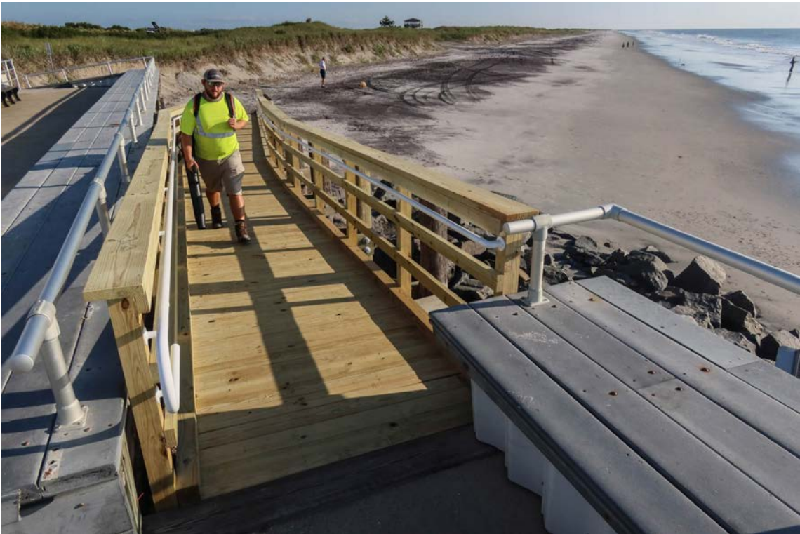
The rebuilt ramp at the north end of the Brigantine is open and gets a blow-dry from Brigantine Public Works on September 4th, 2026. (Photo by Sean Kardon).
