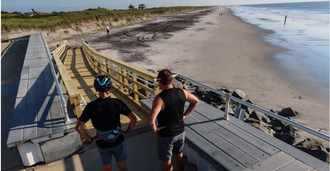
Beachgoers inspect the newly rebuilt ramp at the north end of the Brigantine, which is now open on September 4th, 2026. (Photo by Sean Kardon).
