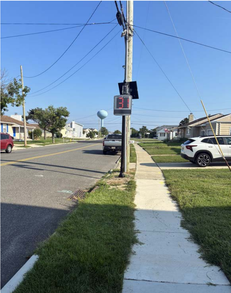
Here’s the new speed radar installed on the 100 Block of North Roosevelt Blvd.
