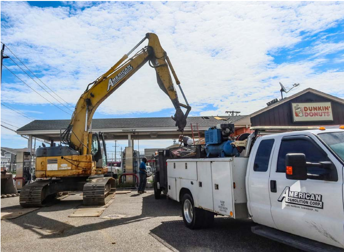
Demolition of the canopy at the closed Gas Station that is connected to the Dunkin Donuts begins at the corner of Brigantine Boulevard and Harbor Beach Boulevard. (Photo by Sean Kardon).
